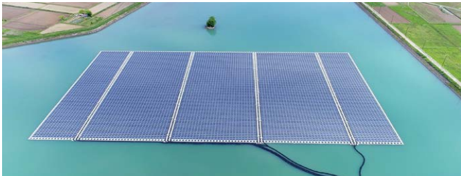
A floating solar array on an irrigation pond in Hyogo prefecture, Japan. Credit: Ciel & Terre International
